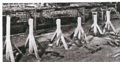
10—Keel form set up and braced ready for keel
